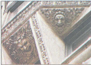
Many of the building's terra cotta pieces have been restored or replaced.
